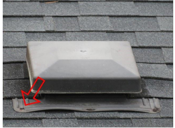
Flashing/Valleys: Views of exposed nail head on vent flashings
