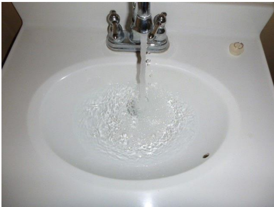
Guest Bathroom: View showing the sink filling up when running the faucet
