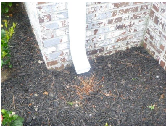
Gutters/Down Spouts: View showing missing splash blocks/extension hoses at the end of downspouts
