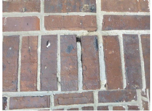
Walks / Steps: View showing the deteriorated mortar joints located between bricks on steps
