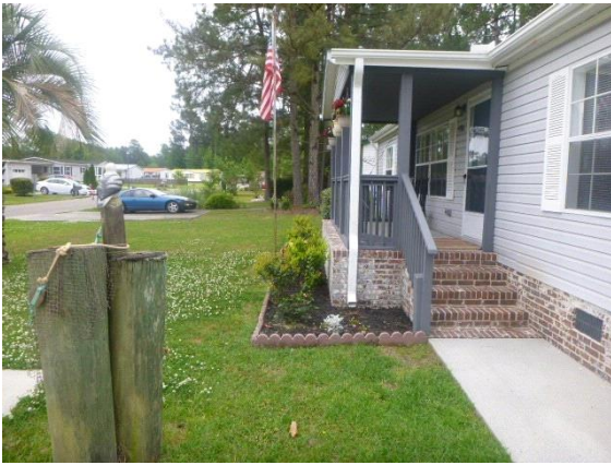
Grading / Drainage: View of front property and grading
