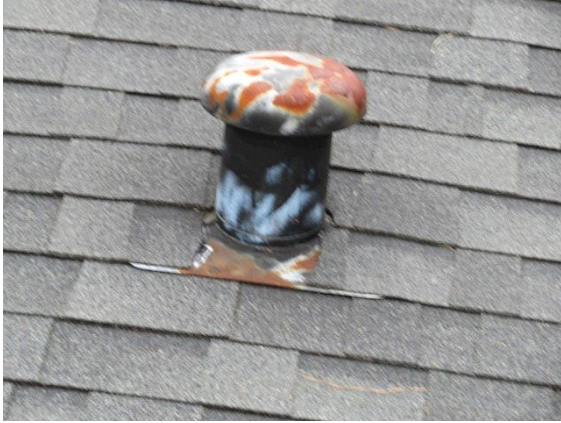
Flashing/Valleys: Views of rusted caps/flashing on vents
