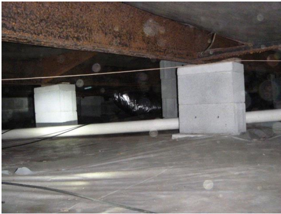
Interior Foundation: View of concrete block piers located in the crawl space
