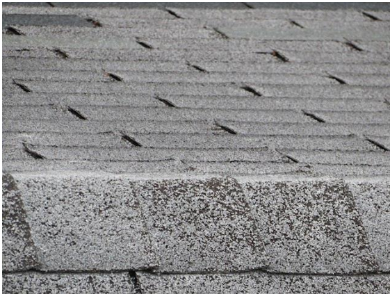
Garage/Carport: Views of excessive granular loss on garage roof shingles
