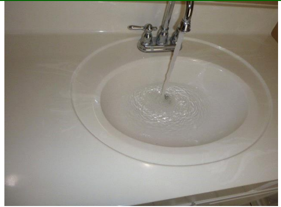
Master Bathroom: View showing the sink filling up when running the faucet
