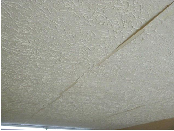
Garage/Carport: View of failing drywall tape on garage ceiling
