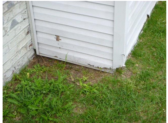
Exterior Surface: View of damaged vinyl siding and trim at base of vinyl chase
