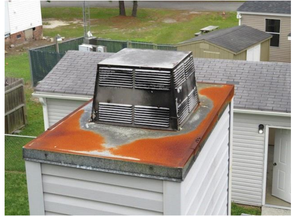
Chimney: View of rusted metal chimney cap
