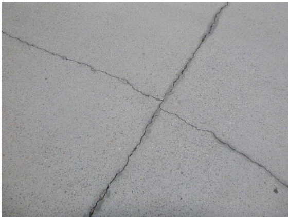
Driveway: View of cracks located in concrete driveway
