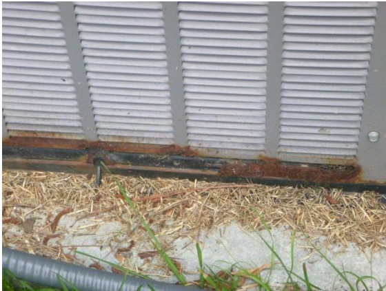
Cooling: View of rust at base of HVAC cover
