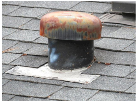
Flashing/Valleys: Views of rusted caps/flashing on vents
