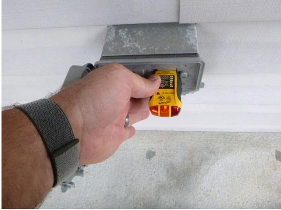
Exterior Surface: View of GFCI receptacle with reversed polarity
