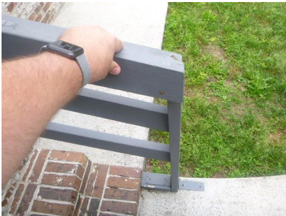
Walks / Steps: View of loose handrail located on the rear steps
