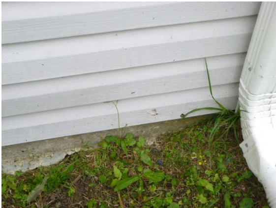
Garage/Carport: Views of damaged vinyl siding and trim on garage exterior
