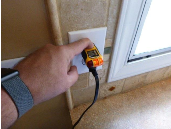
Kitchen: View of kitchen wall receptacle that is not GFCI protected
