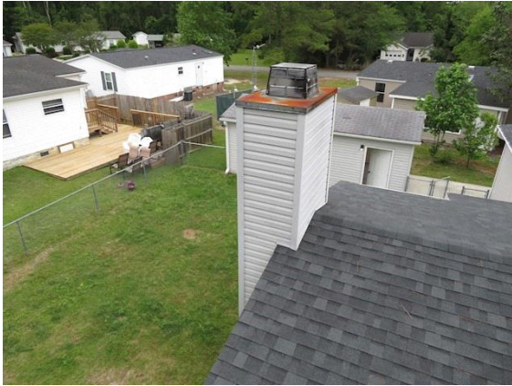
Chimney: Overall view of chimney
