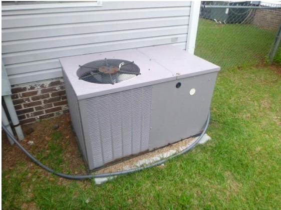
Cooling: View of HVAC package unit located on the back side of the house
