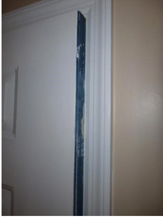
Exterior Doors: View of front entry door hitting frame when closing
