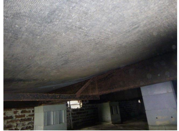
Under Floor Framing & Support: Typical view of black plastic vapor barrier installed on the underside of floor joists
