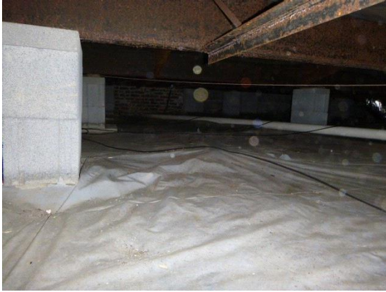
Under Floor Framing & Support: Views of I beam resting on block piers
