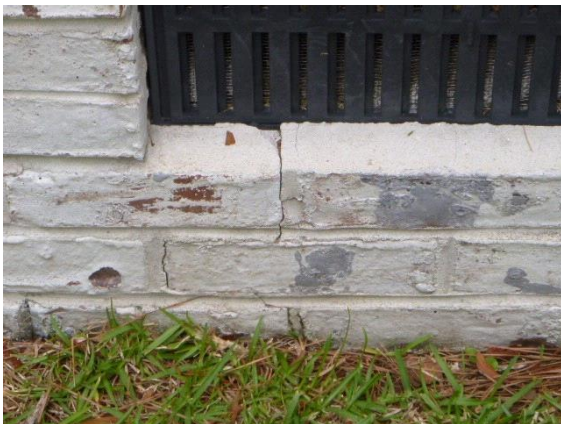
Foundation - Slab: Views of cracked mortar below crawl space vents
