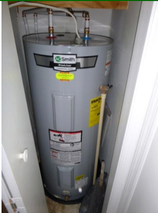
Water Heater: Overall view of water heater located in master bathroom closet
