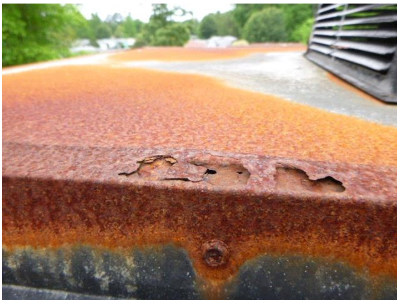
Chimney: View of rusted metal chimney cap
