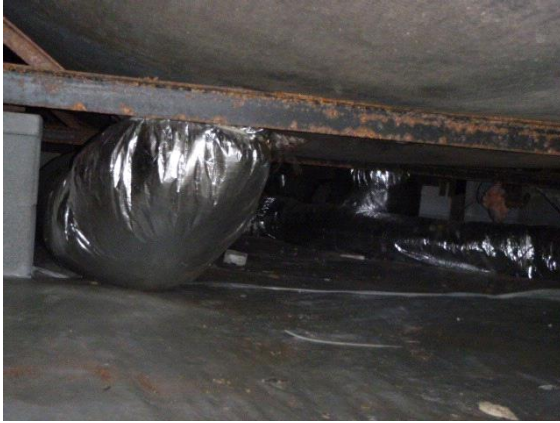
Crawl Space: View of HVAC ductwork laying on the ground
