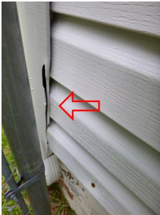
Exterior Surface: View of cracked vinyl trim
