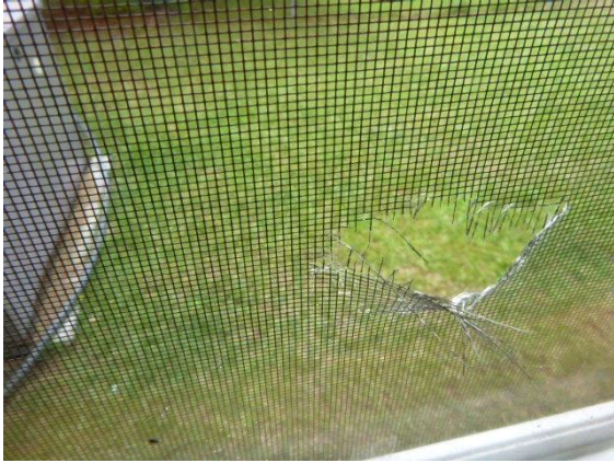
Family Room: View of hole in family room window screen
