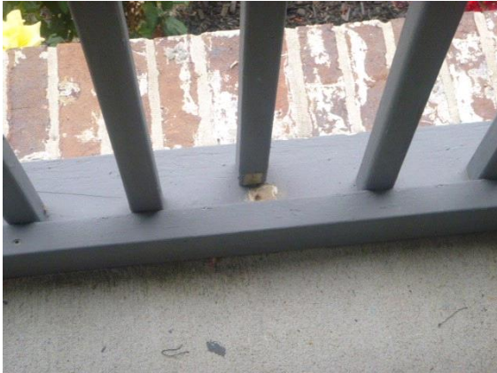
Porches / Stoops: View of loose baluster on front porch
