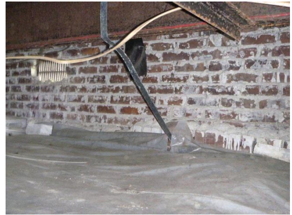
Interior Foundation: Typical view of metal tie down straps located in the crawl space
