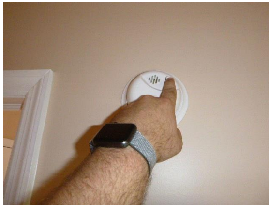
Electrical: All smoke detectors were checked and are operational
