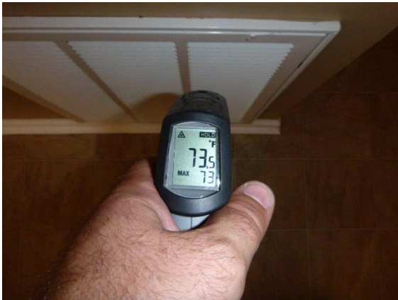
Heating: View of return air temperature using a digital thermometer in the heating mode
